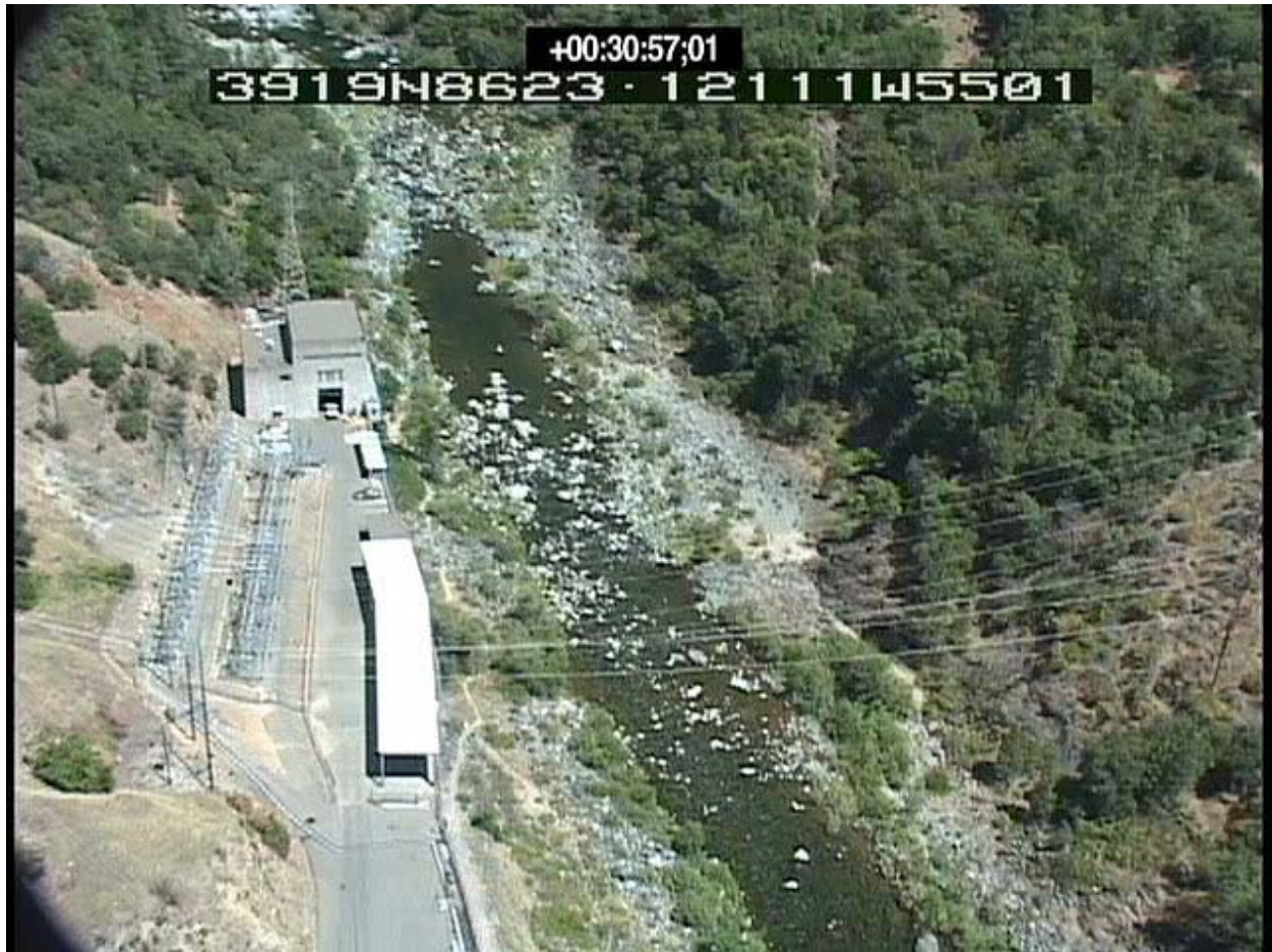
Figure 3.0-6. Yuba River MNYRR, Section 1 at RM 34.0, looking upstream from New Colgate Powerhouse.
