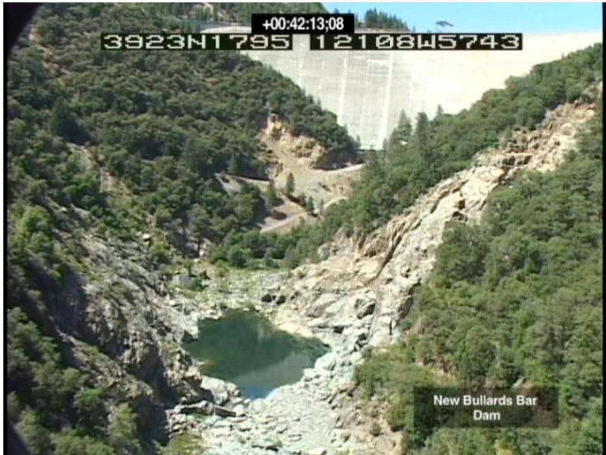
Figure 2.0-17. North Yuba River NBBDR, Section 3 near RM 2.0, looking upstream at New Bullards Bar Dam. Spillway pool requires boat to cross.
