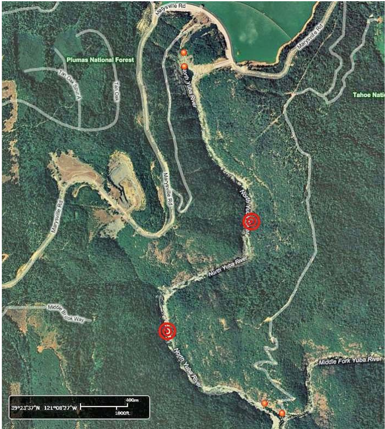
Figure 2.0-3. North Yuba River – New Bullards Bar Dam Reach: overview aerial image. The approximate extent of the March 2011 reconnaissance areas are demarcated by red dots (two short sections). Concentric red circles indicate approximate extent of inaccessible middle section of reach (with boat and at low flows).
